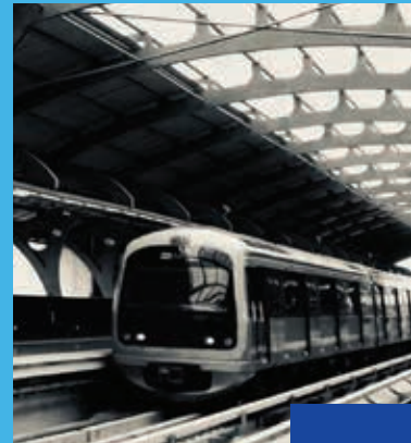
MUMBAI ELEVATED METRO
