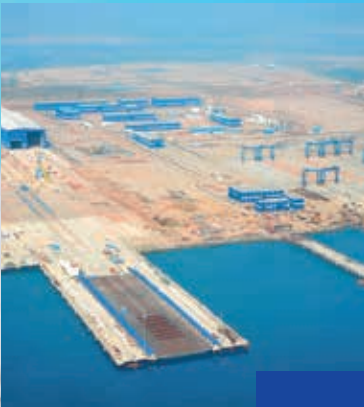
CHENNAI PORT (L&T AND ECC GEO STRUCTURE), TAMIL NADU
