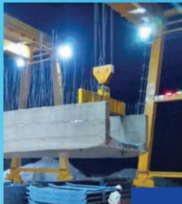
YETTINAHOLE AQUEDUCT PROJECT, BANGALORE
